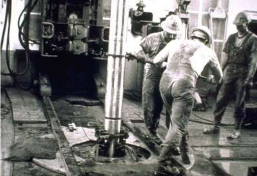
Figure 25. Two Drill Collars made up. Note that alignment is difficult, and the environment is not dry/clean [5].
